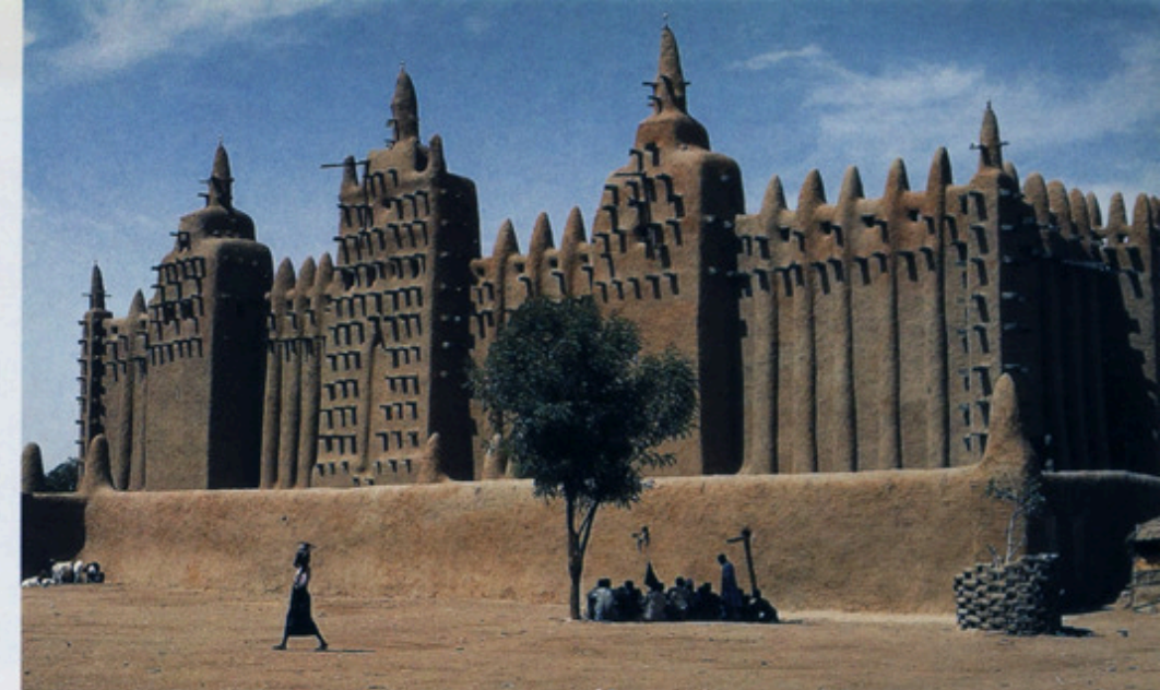
Adobe-built houses and the mosque of the city of Djenné, Mali. The mud buildings are two storeys high, and the mosque is the largest mud-built structure in the world.
