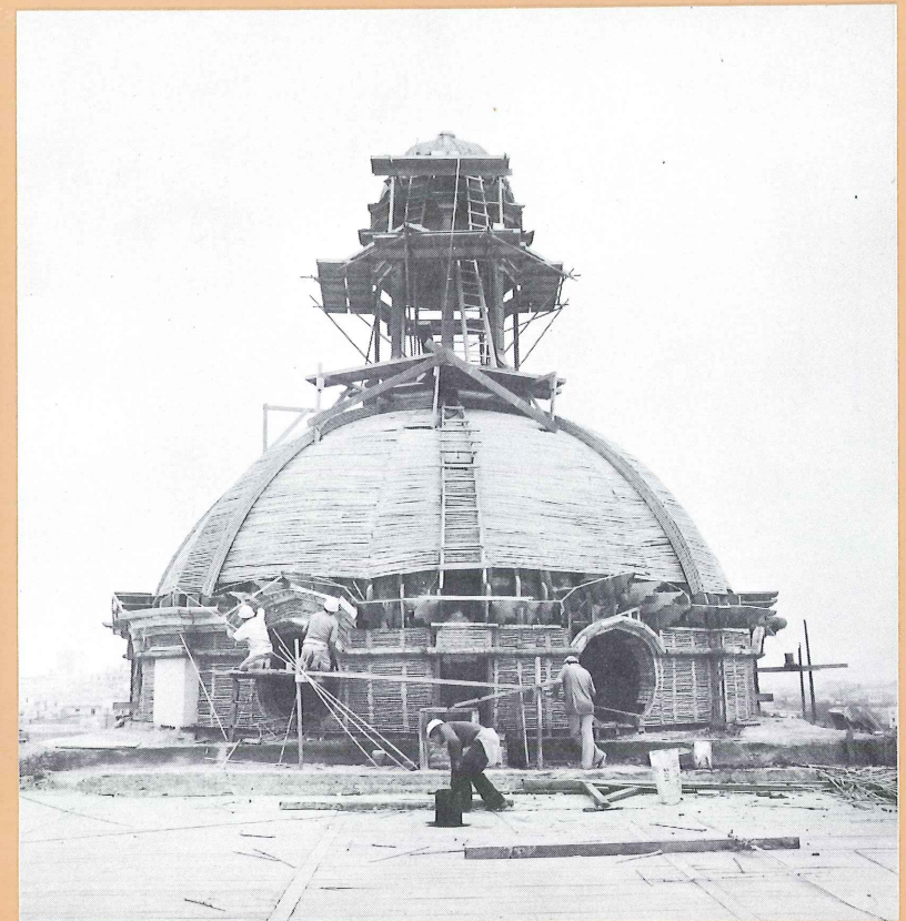
Cúpula de madera y caña / Dome made of wood, cane and mud. San Francisco, Lima, Perú.
