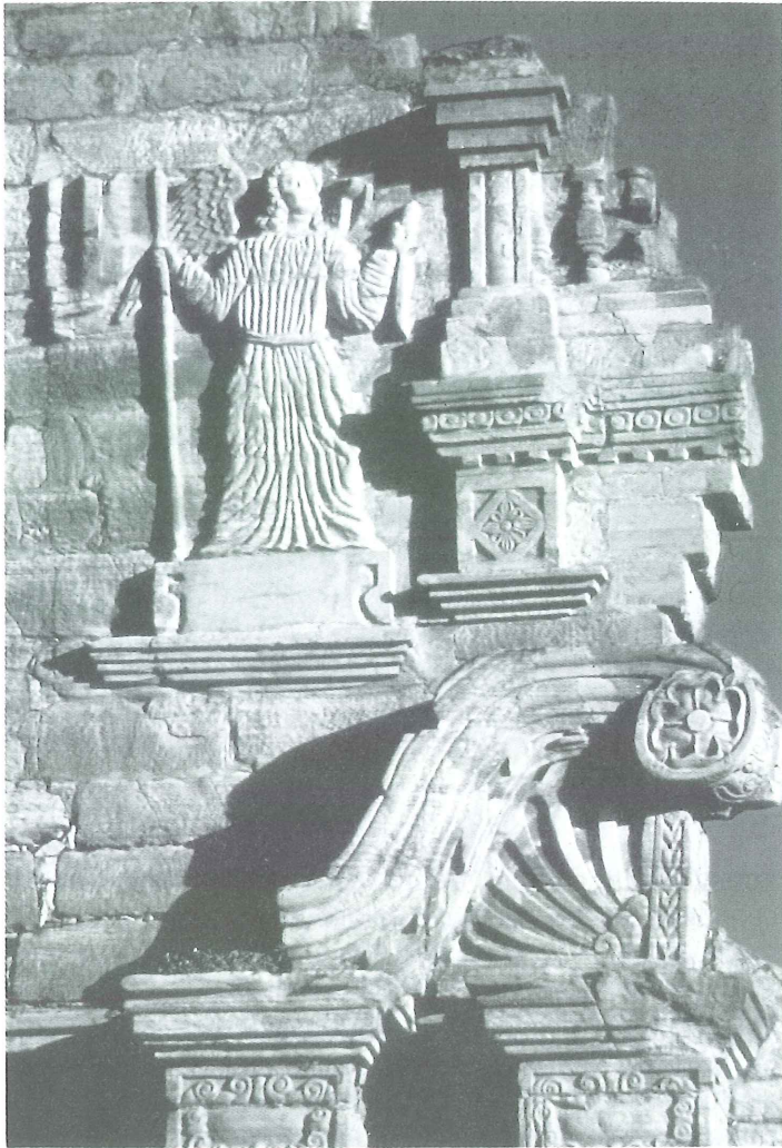
Detail of stonework at San Ignacio Mini, Argentina. Photo: Hannquin
