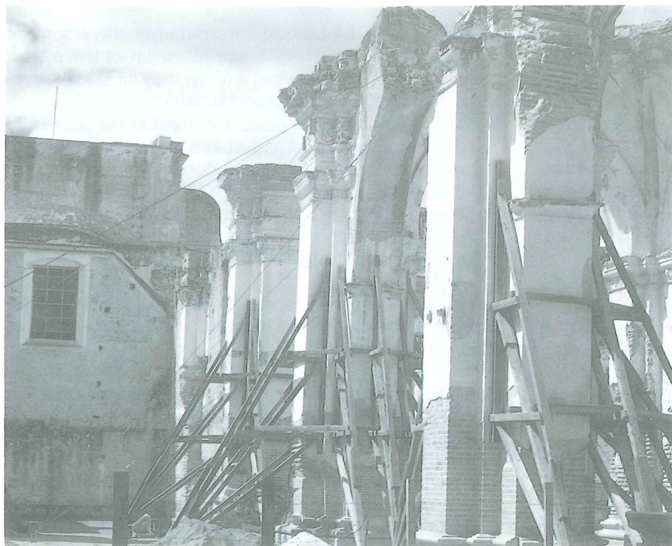
Anti-seismic restoration in Antigua, Guatemala.
