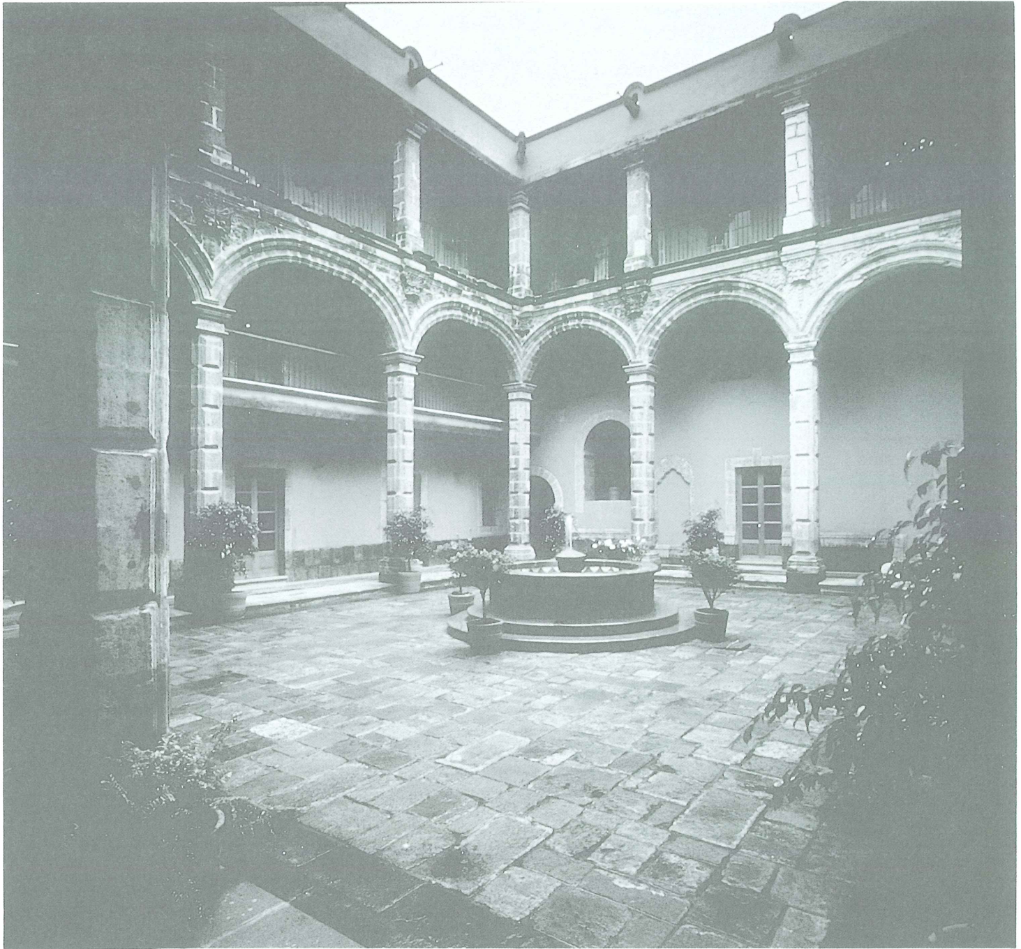
Courtyard restored through fiscal incentives of the Integral Renewal Programme in Mexico City.
