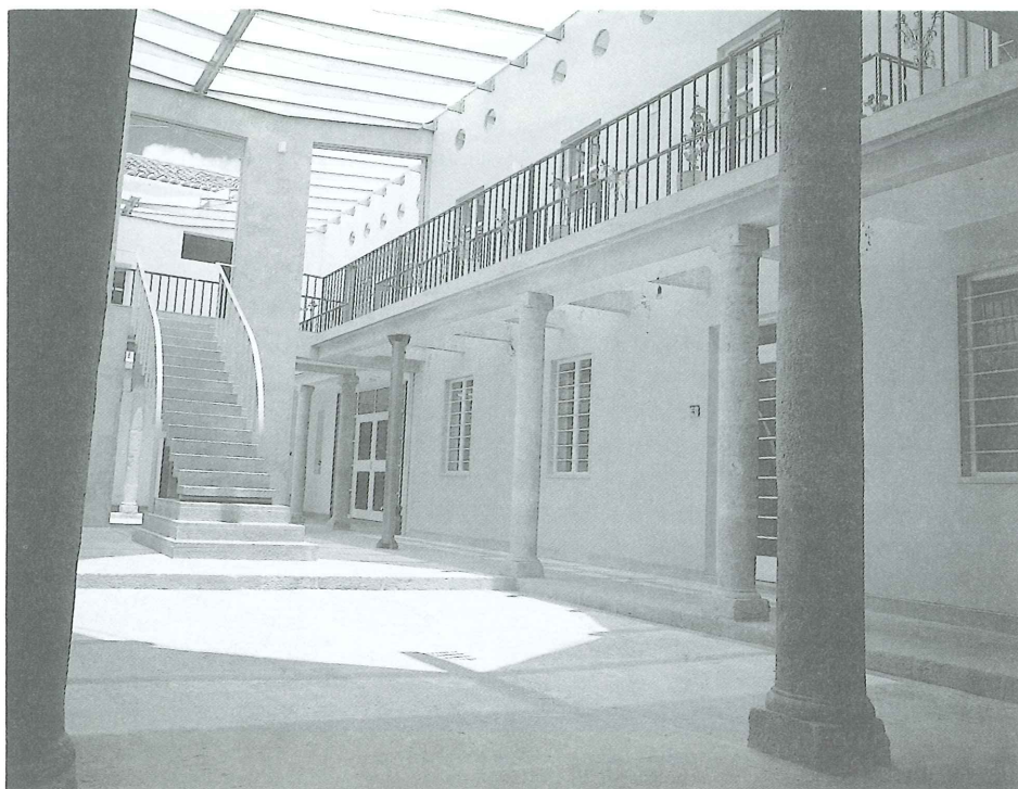
Interior of Quito's house of seven patios after restoration work. Photo: F. Salazar
